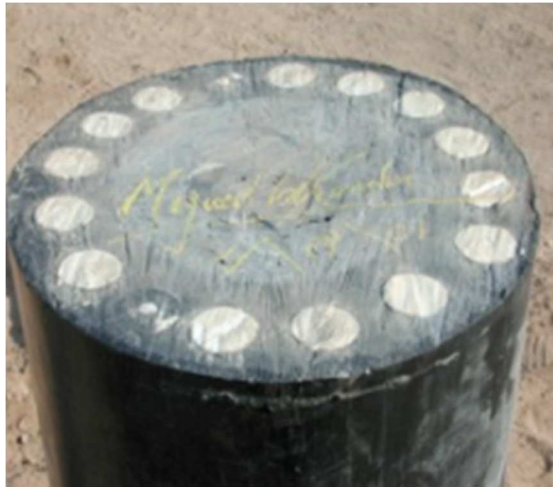
Figure 3 Plastic marine piling reinforcement.
